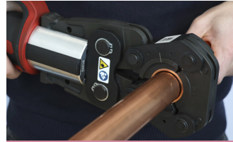
3. Complete the joint with the press tool
